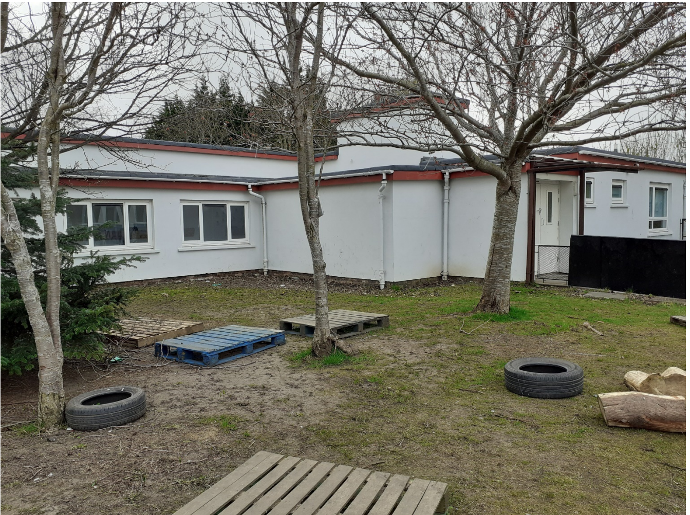
Photograph of Brunstane Primary School nursery building external walls after enhancements
