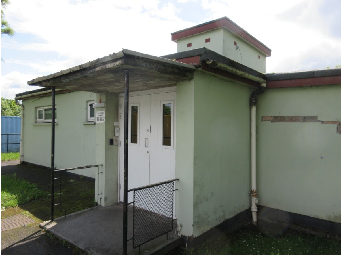
Photograph of Brunstane Primary School nursery building main entrance before enhancements
