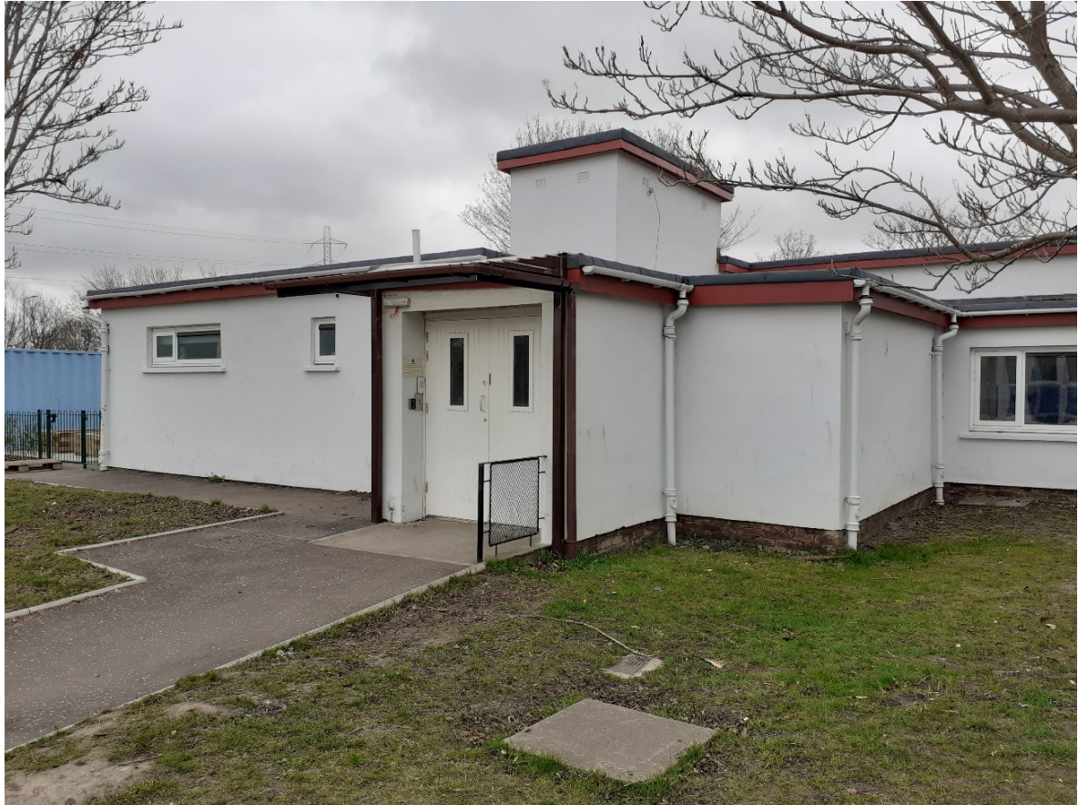
Photograph of Brunstane Primary School nursery building main entrance after enhancements
